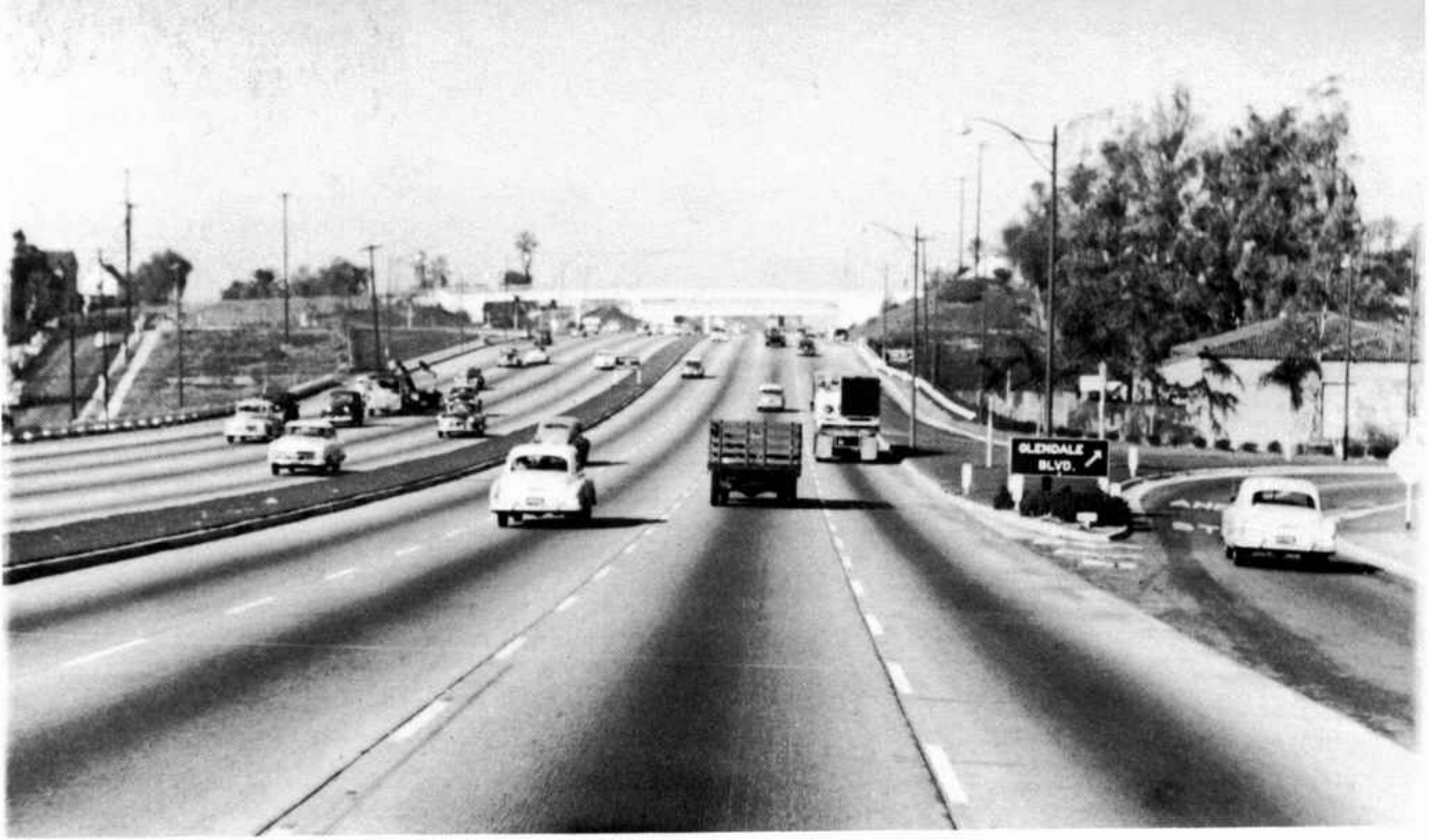
Looking west on the Hollywood Freeway.
