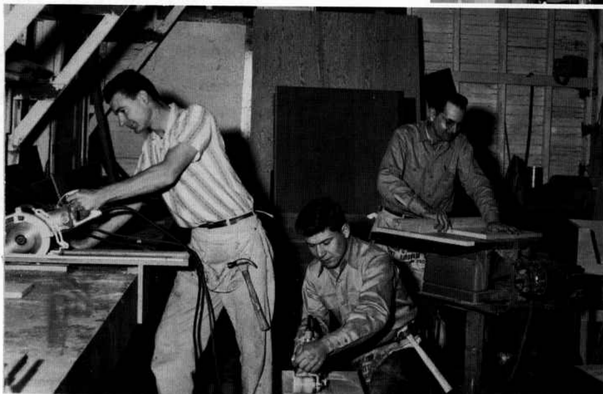
A steady stream of office equipment, bookshelves and student desks flows from our cabinet shop and the tools of Bill Rapp, Sidney Rumpel and Homer Jamison.
