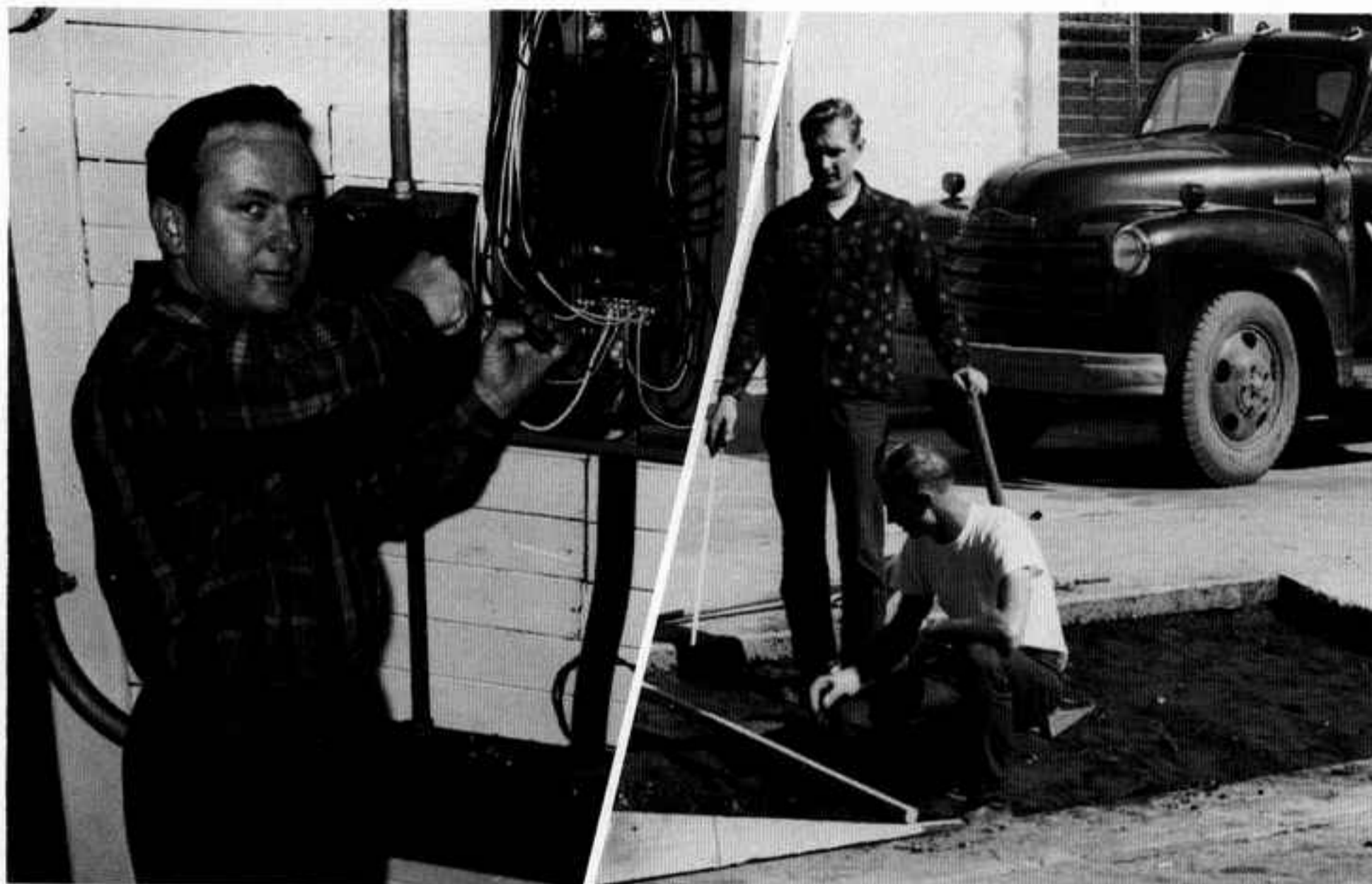
Left —The mysteries of an electrical circuit are untangled quickly by Edmund Smith. Right —Supervision in the Construction and Maintenance Department by Dennis Glover means profitable employment for students and profitable employees for the College.
