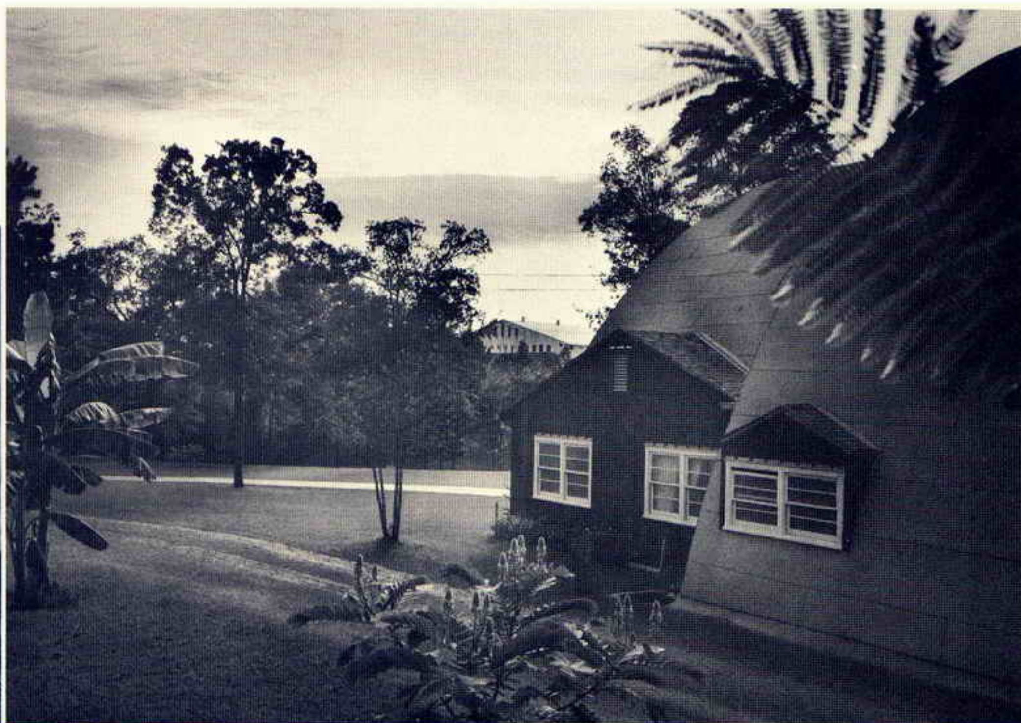
A view of progress—the dining hall in a foreground of tropical plantings with the newly constructed tabernacle in the distance.
