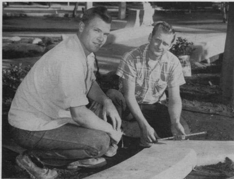
Many projects keep our construction and maintenance crew busy. Dennis Glover, Construction Foreman (right) and Max Kuhlmann, assistant, look over the latest project.
