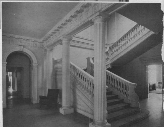
Above: A view of Memorial Hall just inside the entrance gate. Center: The Entrance Vestibule. Right: The Grand Hall.
