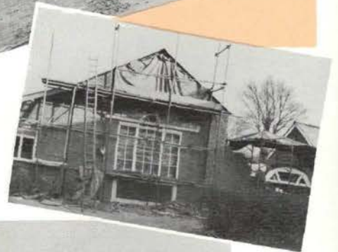
Well along in its construction.
