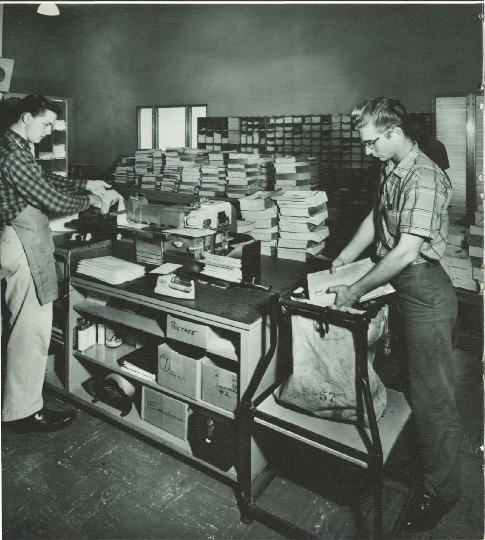
Hundreds of letters hourly pour from this postage meter which seals the envelopes and affixes the proper amount of postage.
