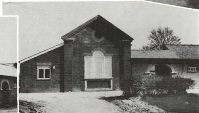
The large window will be stained glass. Below this, a large inscription plaque will be mounted.
