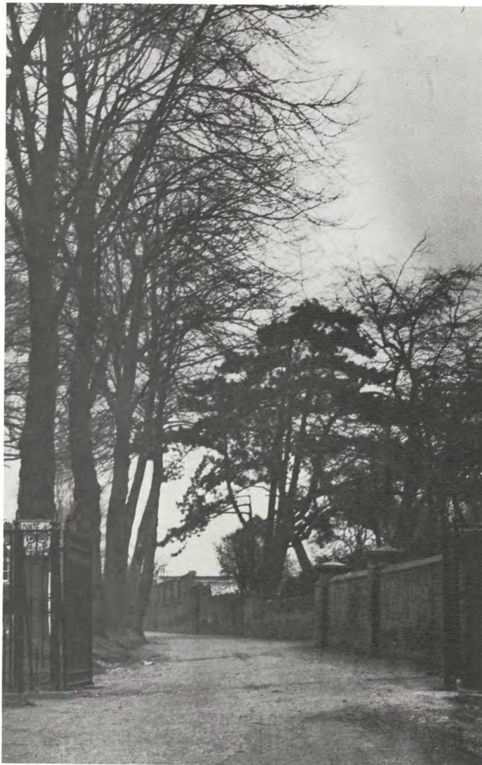
Drop Lane Gates. At present this is being used as Main Entrance to grounds.
