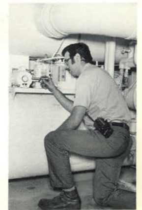
Scott Warner works on an air conditioning unit.
