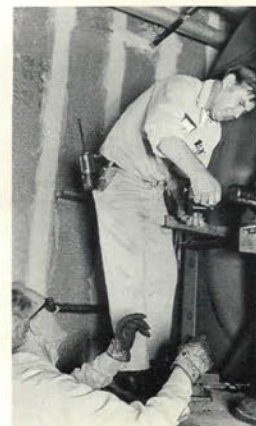
Ken Zlab and Jim Wendt check the air conditioning in the basement of the Hall of Administration.
