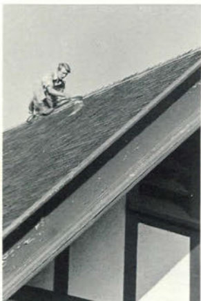
Carpenter Joe Shuster works on a roofing job.
