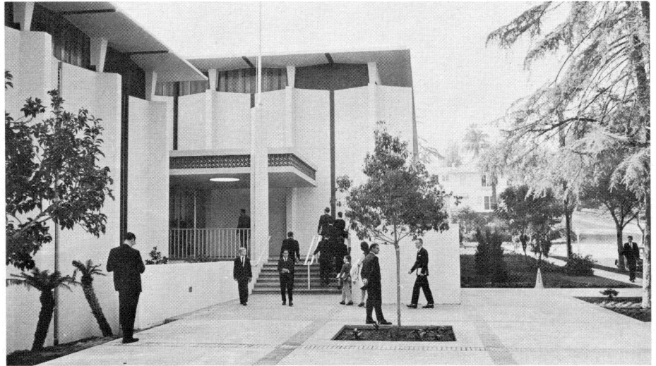
FRONT ENTRANCE —Daylight view of spacious main entrance to new gymnasium. Concrete work and landscaping were all done by Ambassador personnel.
