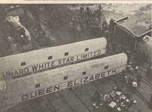
The docks at Southampton, England.
