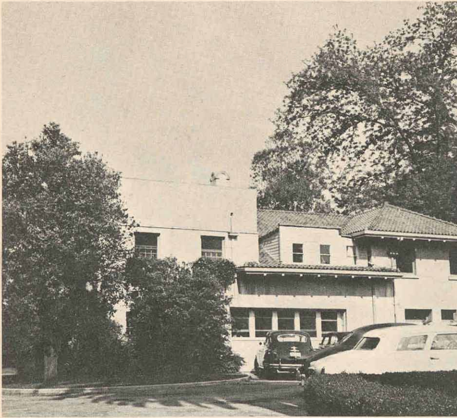
View of the Administration Building as it appeared in 1947. It now contains many of the executive offices of the College and Work.
