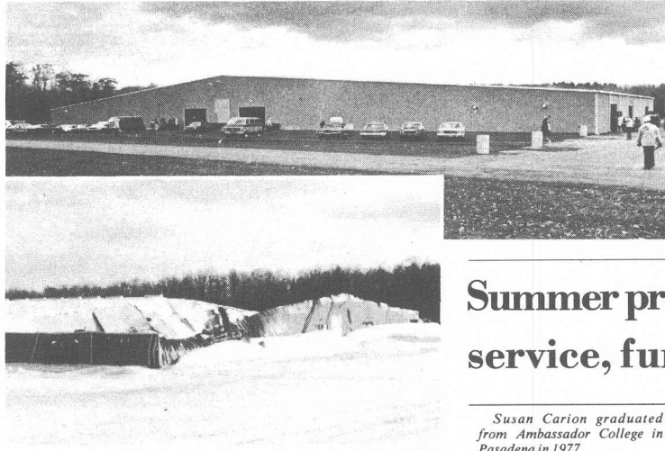
BEFORE AND AFTER — Members exit the repaired Church building in Mount Pocono, Pa., after 1981 Feast services, top photo. Above, the building following the January, 1978, storm. [Top photo by Michael Snyder]
